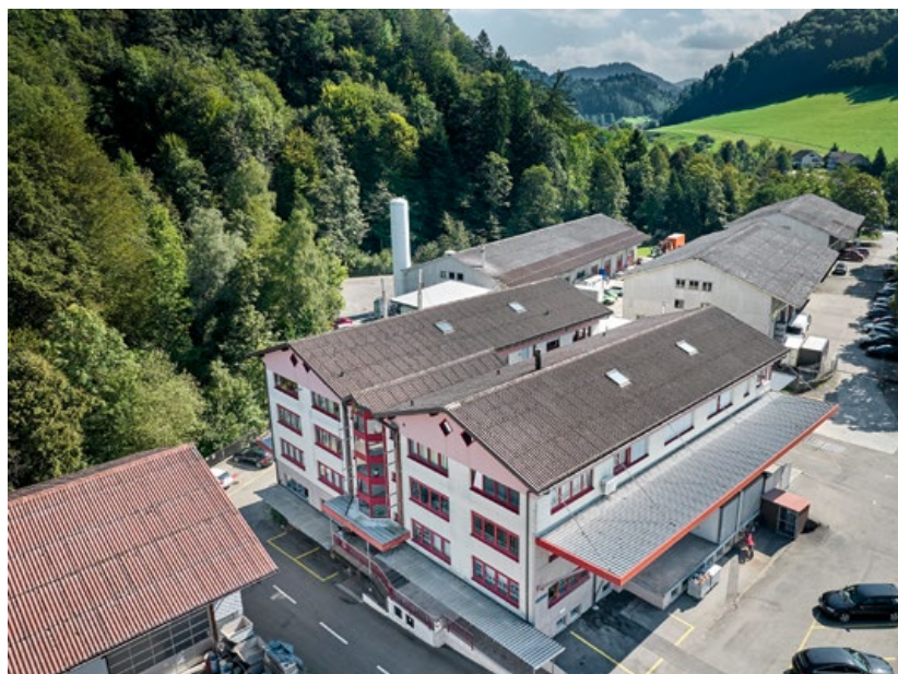
Fig. 1 Buildings at the Parmaco MIM facility in Fischingen, Switzerland (Courtesy Parmaco)
