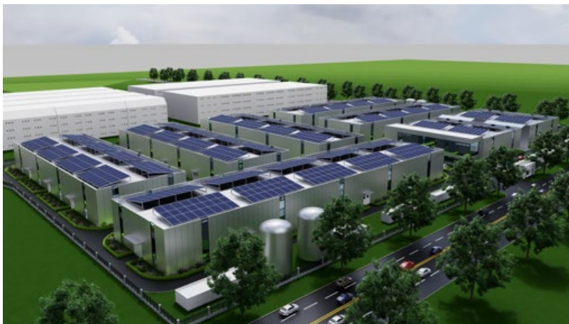
CNPC is constructing an R&D facility in California to support its North American customers (Courtesy CNPC Powder)
