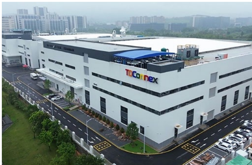
TDConnex's new Xiamen 6 facility will significantly expand its MIM capacity and boost its production of micro-components for consumer electronics (Courtesy TDConnex)
